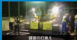
舗装の打換え
