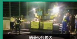
舗装の打換え
