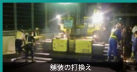
舗装の打換え
