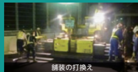
舗装の打換え
