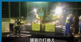
舗装の打換え
