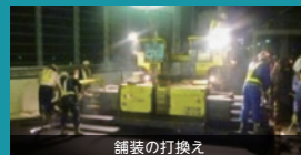
舗装の打換え
