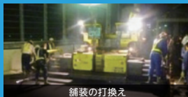
舗装の打換え
