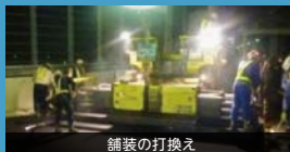
舗装の打換え
