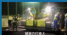
舗装の打換え
