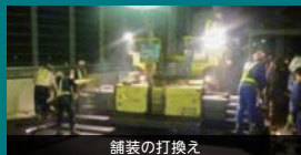
舗装の打換え
