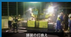
舗装の打換え
