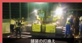
舗装の打換え
