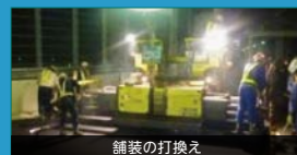
舗装の打換え
