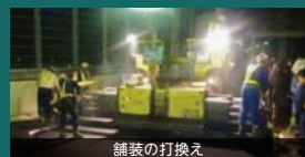
舗装の打換え
