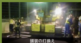
舗装の打換え
