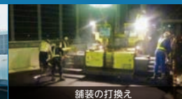
舗装の打換え
