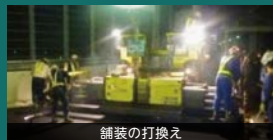
舗装の打換え
