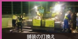
舗装の打換え
