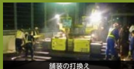
舗装の打換え
