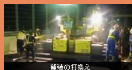
舗装の打換え
