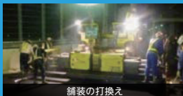
舗装の打換え
