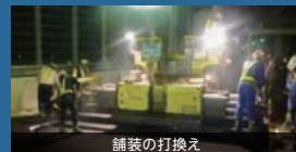
舗装の打換え
