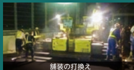
舗装の打換え
