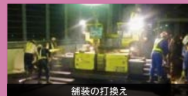
舗装の打換え
