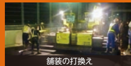
舗装の打換え
