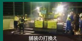
舗装の打換え
