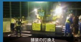
舗装の打換え
