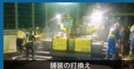
舗装の打換え
