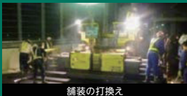
舗装の打換え
