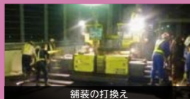
舗装の打換え
