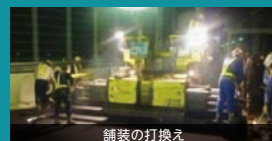
舗装の打換え
