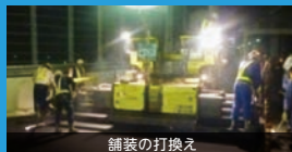
舗装の打換え
