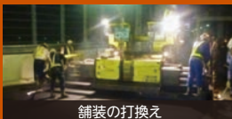
舗装の打換え
