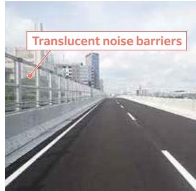
Installation of noise barriers and ground-facing sound-absorbing panels
