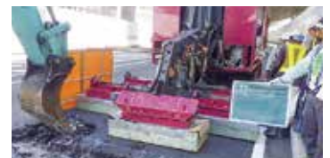
IH pavement removal in operation
