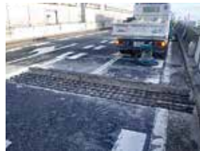
Completion of bar arrangement
